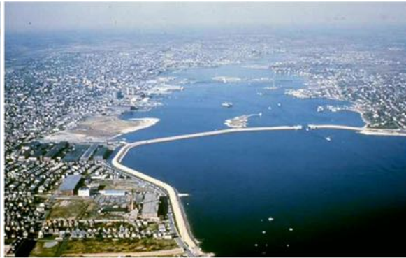
New Bedford Harbor, MA 1.8 miles long with single 100ft wide gate, $ 200 million
