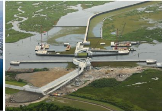
Intracoastal Waterway, New Orleans 1.8 miles long, $1.24 billion
