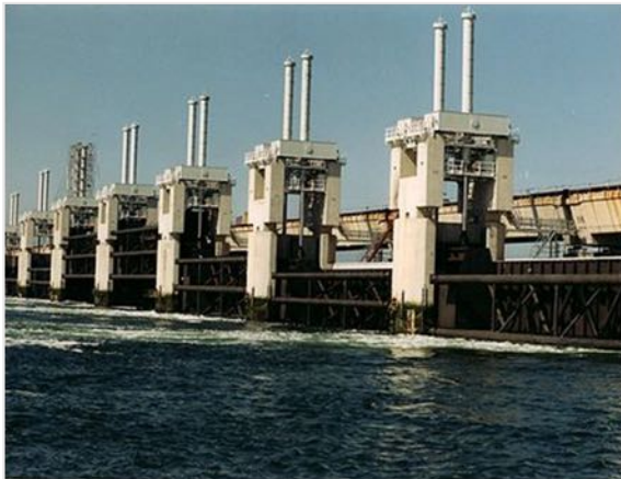
Drop gate lowered into defense position, prevents navigation
