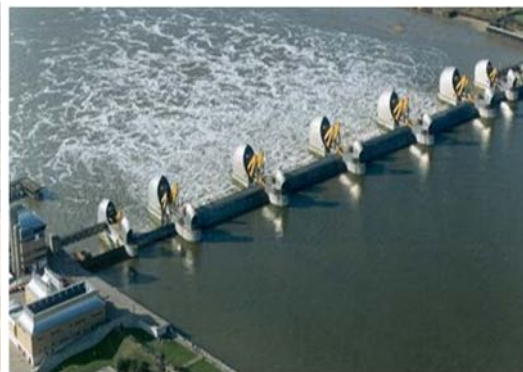
Thames Barrier, London 1,700ft long with 4 no. 200ft wide and 6 no. 100ft wide gates, $ 2.59 billion
