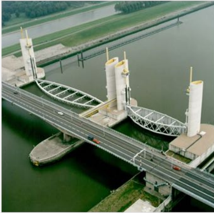
Lift gate lowered into defense position, significant air draft to allow navigation
