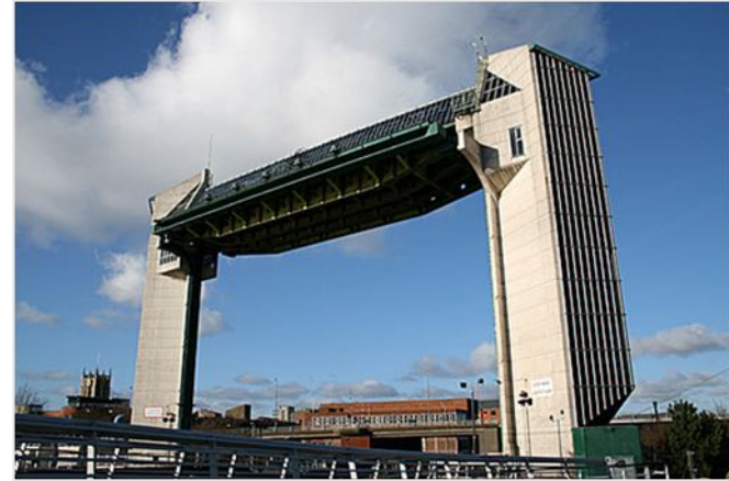
Lifting gate lowered into defense position, significant air draft to allow navigation
