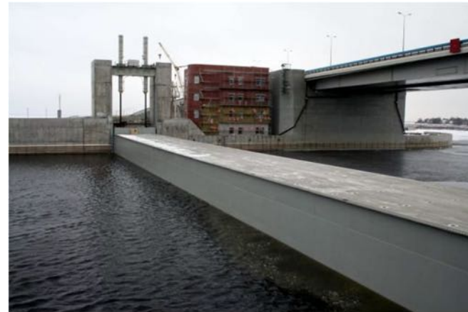
Lift gate raised into defense position from its seabed chamber
