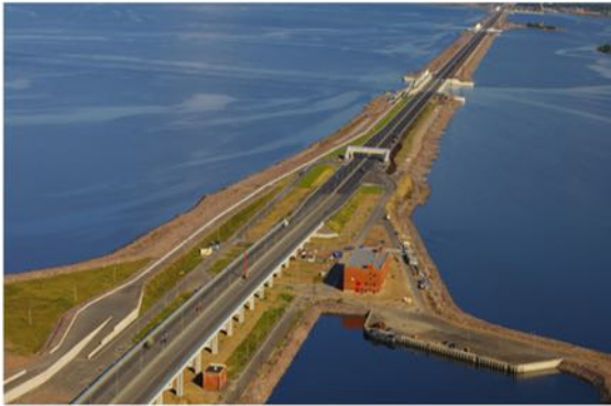
St. Petersburg, Russia 16 miles long with 650ft wide sector gate and 340ft wide lift gate, $ 6.4 billion
