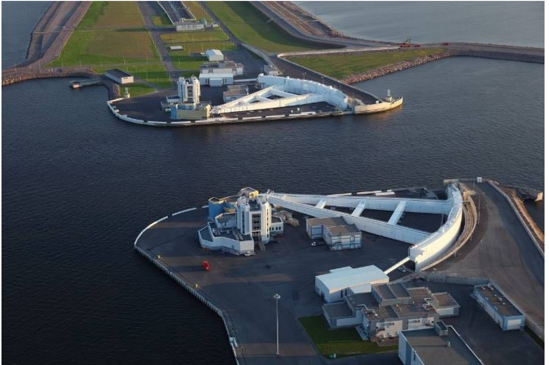
Taintor gates in open position at the St Petersburg storm barrier system
